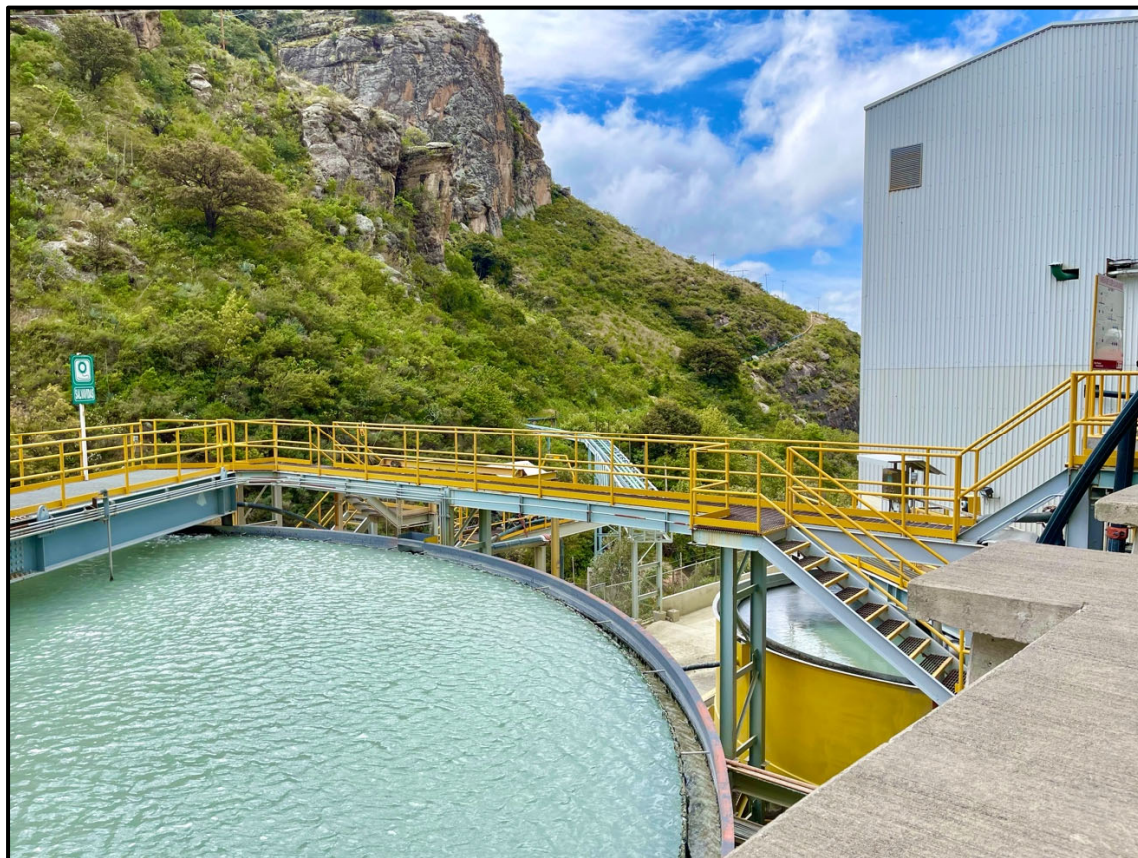
Settling tank at El Cubo
